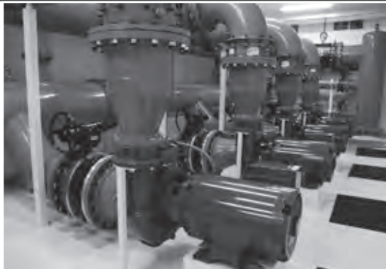
Booster Pump Systems
